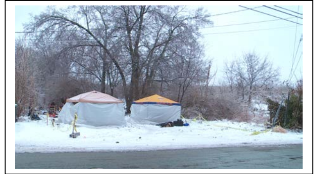
Figure 4: Fieldwork at the same site after demolition on 12/17/2010.
