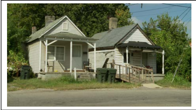
Figure 3: Shotgun homes at 710 and 712 DeRoode before demolition on 11/17/2010.
