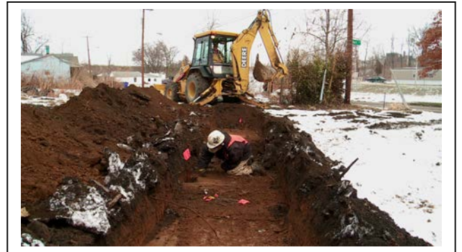
Figure 8: Flagging wood-pier posts uncovered from subsurface excavations on 12/29/2010.
